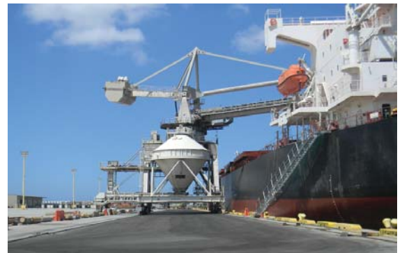
Coal is being unloaded at KBPH Pier 6 by a bulk unloader, which is then carried by a conveyor system to the AES plant.
